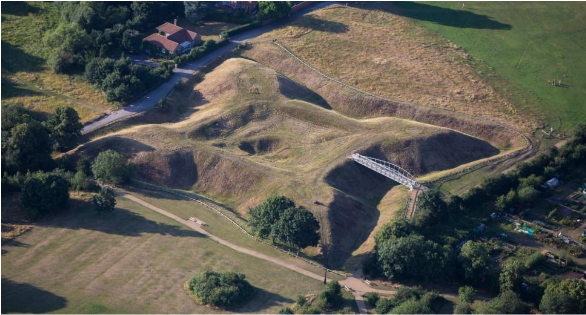
Plate 1: Newark Sconce: an example of a large metal bridge crossing earthworks
