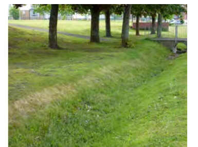
Swale drainage features
